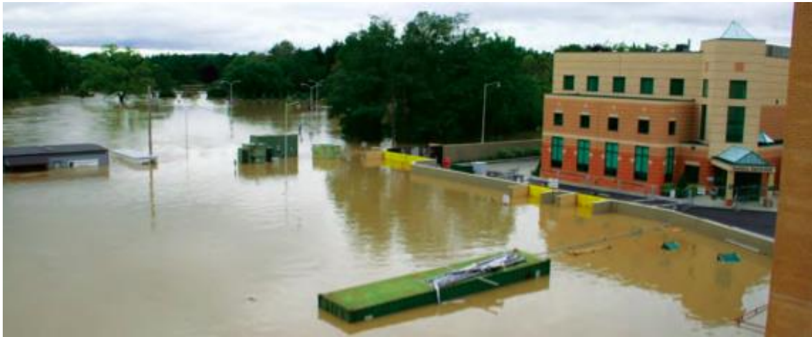
Lourdes Hospital from 2011 flood (FEMA)
