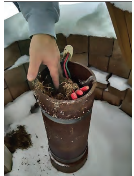
Broken well cap with mouse nesting material in Madison County, New York.
