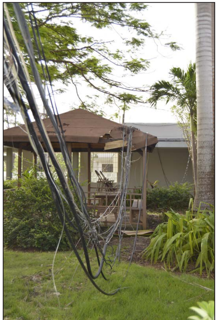
FIGURE 1. Disruption of electrical grid powering the Puerto Rico Department of Health laboratories caused by Hurricane Maria — San Juan, Puerto Rico, September 2017*
