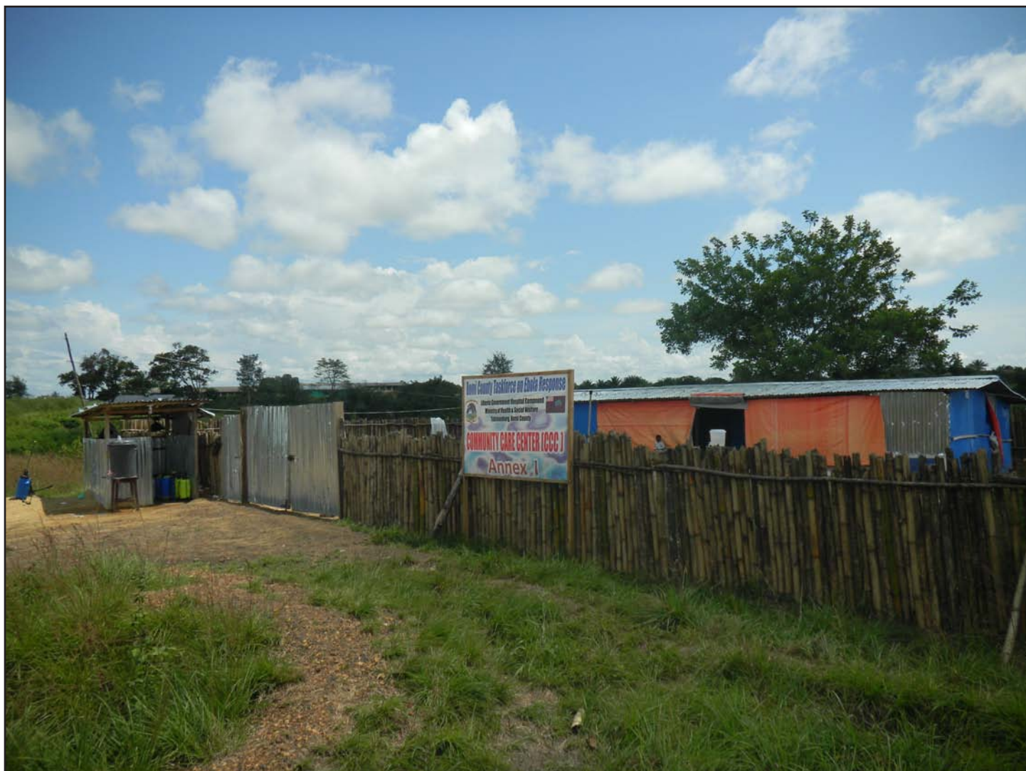
FIGURE. Bomi County community care center, Liberia*
