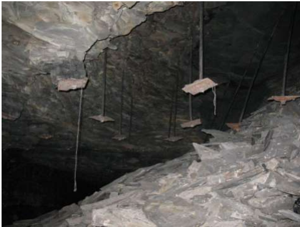
Figure 15: Extreme roof deterioration in moisture-sensitive shale at an Illinois coal mine.
