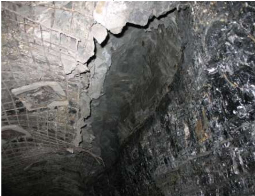
Figure 17: Exposed corners in wide entries can lead to guttering and eventually roof fall.
