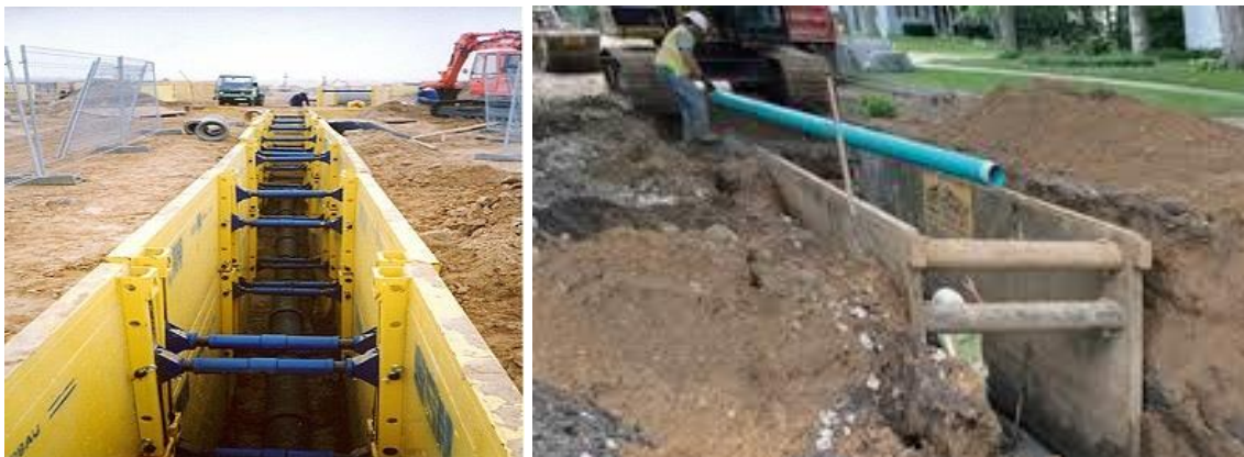
Figure 6. Stock photos of trench shoring (left), trench box (right).
