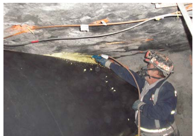
Figure 10. Application of PUR to the perimeter of the Ventstop ® ™ unit.
