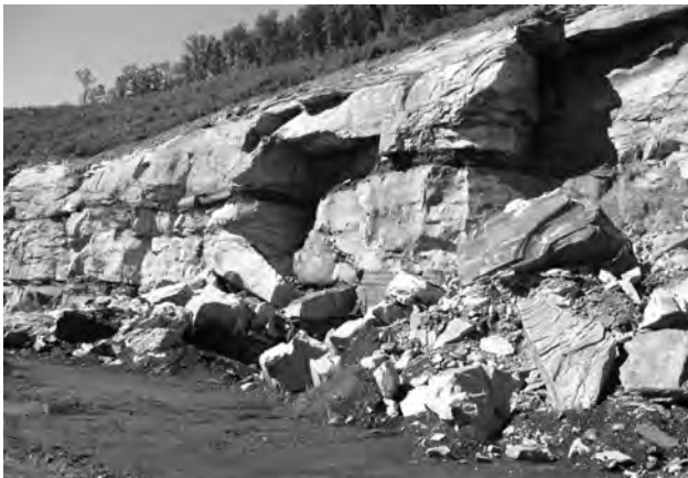
Figure 13. Highwall collapse in multiple seam mining area.
