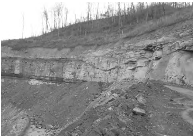
Figure 14. Highwall collapse in multiple seam mining area.
