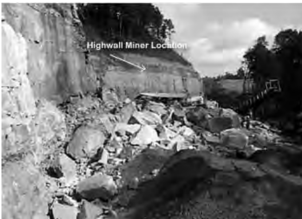
Figure 3 – Highwall collapse resulting in fatality.
