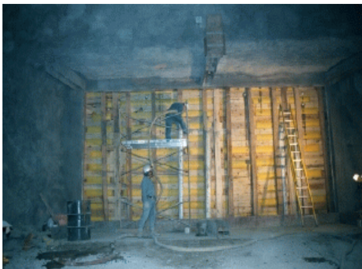
Figure 3. View of mine seal at a late stage in construction.
