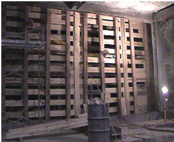
Figure 2. Mine seal form under construction showing posts and cross members.
