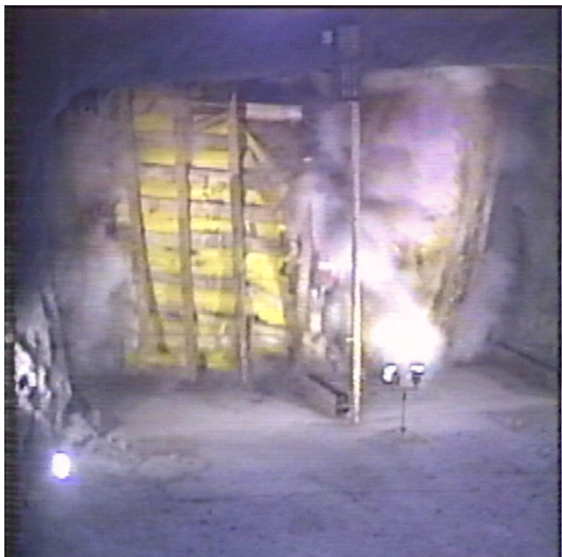
Figure 13. Failure of middle-right side of seal.
