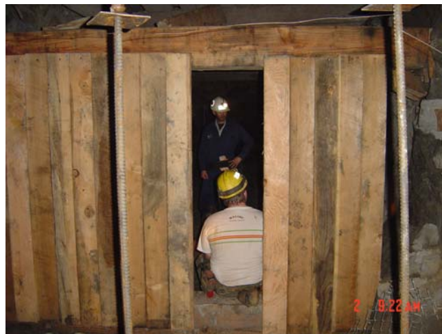
Figure 5. Backfill retaining wall construction.
