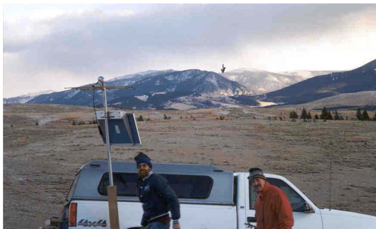
Figure 2. Mission Creek repeater station
