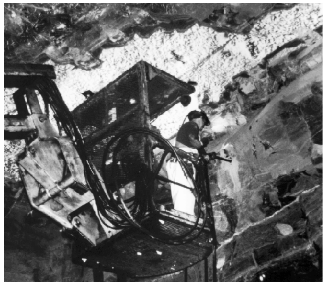
Figure 33.—Explosives being loaded into borehole at Long Ridge Mine.
