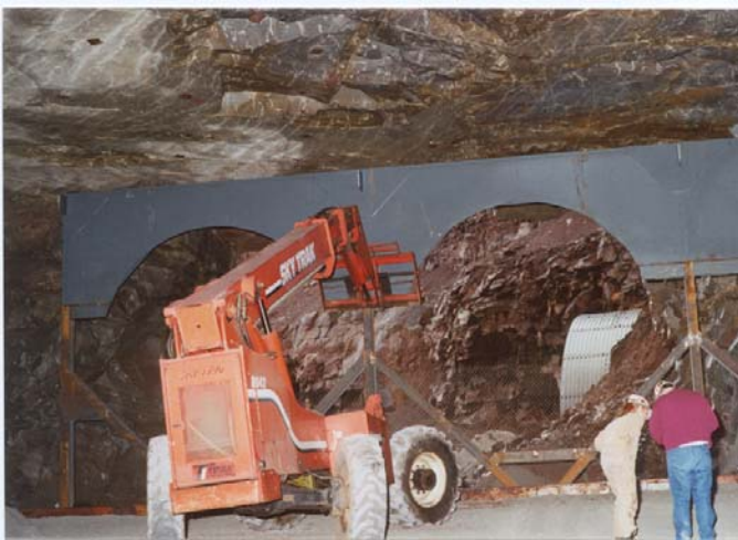
Figure 7. Installation of prefabricated fan bulkhead
