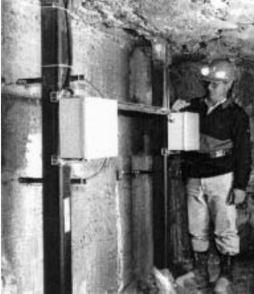
Full-scale, reinforced cementitious seal instrumented with transducers and accelerometers to measure displacement of the seal during an explosion.
