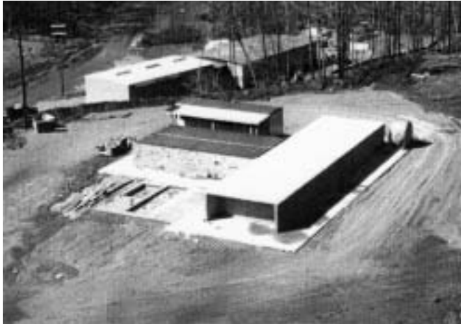
Fire suppression facility at Lake Lynn Laboratory.
