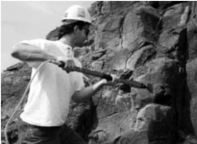
Demonstrating the technical feasibility of a pneumatic scaling tool.
