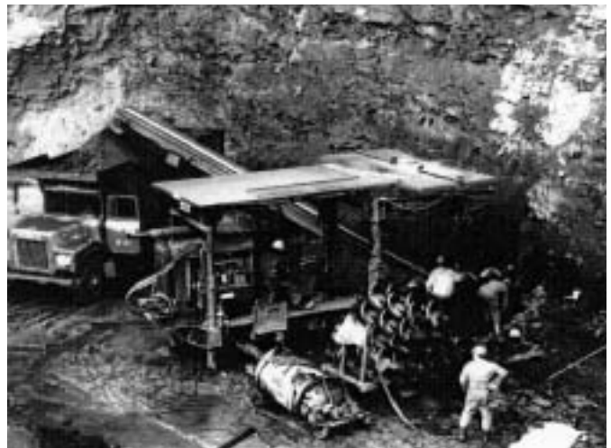
Measuring explosive gas concentrations in augered mining holes using a wireless transmitter.
