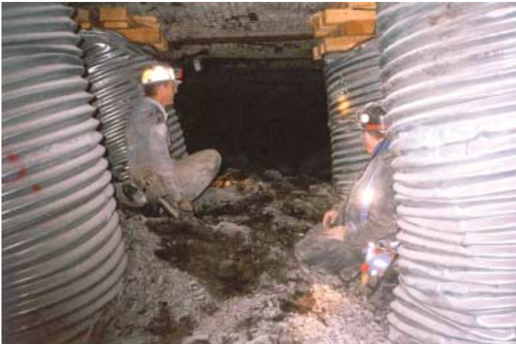
Figure 9. Large amounts of floor heave shown outby the longwall face caused compression of the support which allowed it to develop sufficient load-carrying capacity for roof support in this installation.
