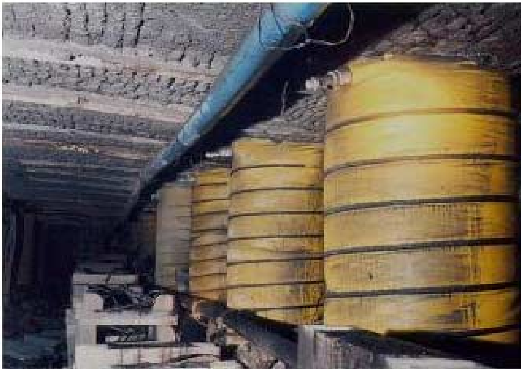
Figure 22. Pumpable support just inby the face showing that the support has not deformed much, indicating that this is primarily a load-controlled environment or that the displacement-controlled activity did not cause more than 1 inch of convergence.
