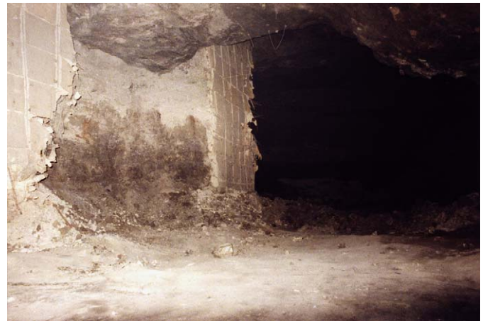
Fig. 13. Stable backfill after pillar extraction.
