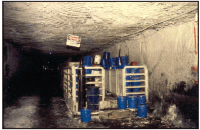
Figure 15.—Underground oil storage area.
