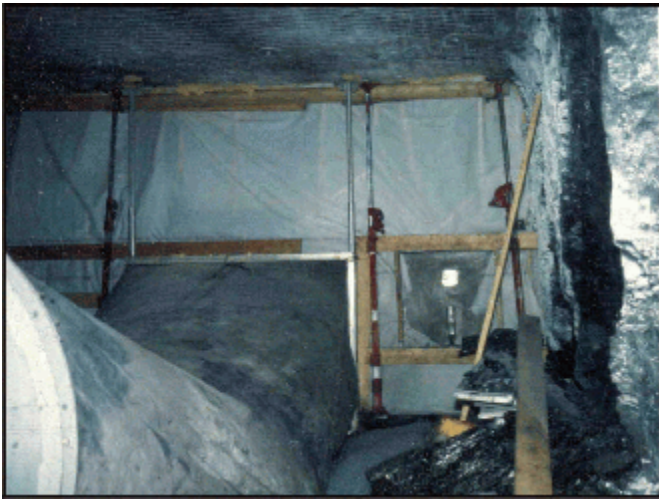
Figure 6.—Erecting a typical mine stopping for a high-expansion foam generator.
