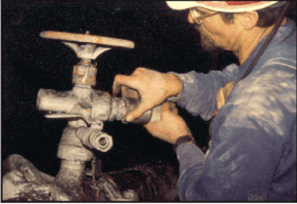
Figure 3.—Inspection of an underground fire hydrant.
