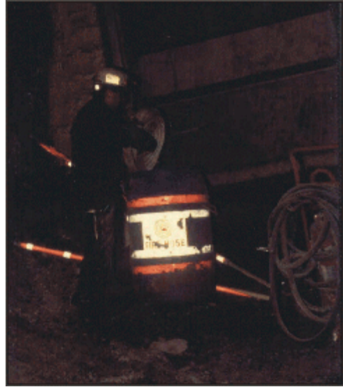
Figure 4.—Underground storage of fire water hose in barrel.
