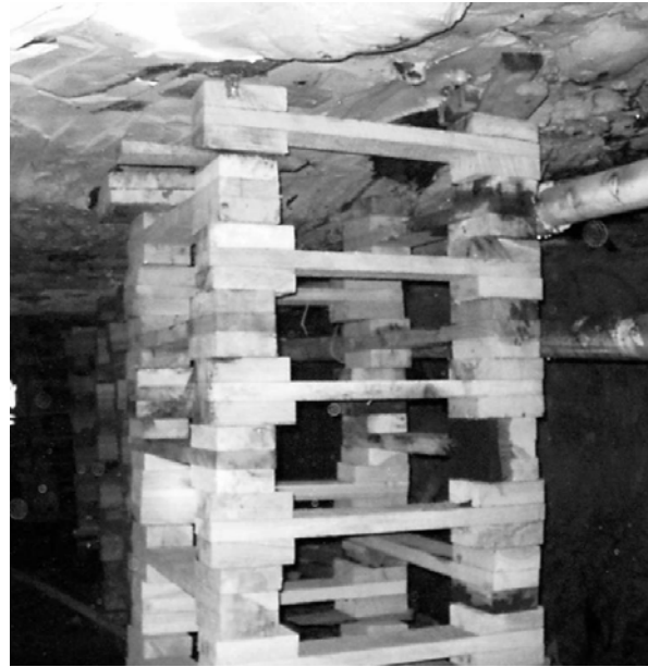
Figure 3. The ATLAS 100 engineered crib installed in the tailgate.
