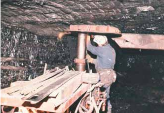
Roof bolter operator under roof canopy during roof drilling.
