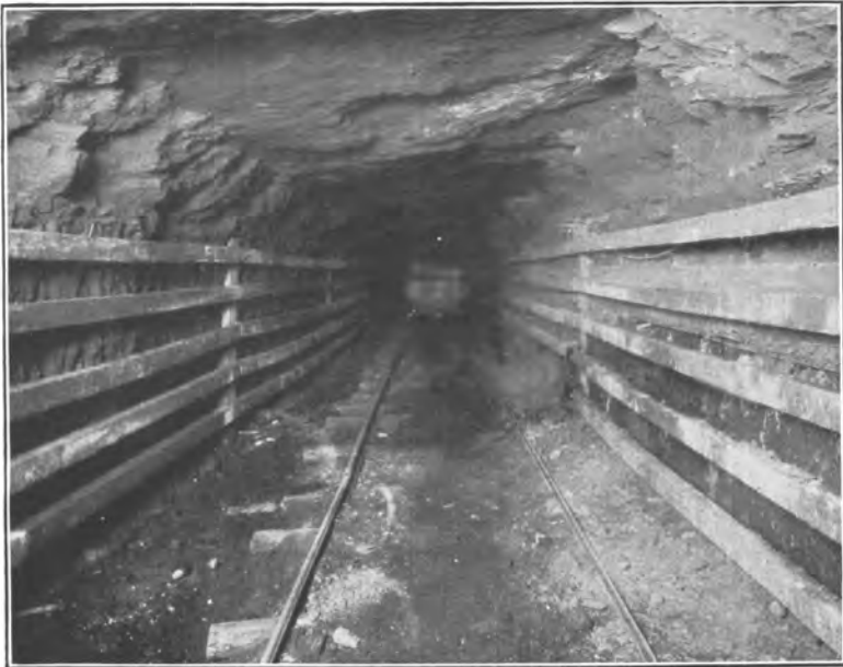
A. DUST SHELVES IN MAIN ENTRY.
