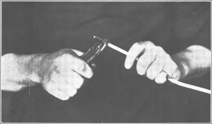
A. CRIMPING DETONATOR ON FUSE.
