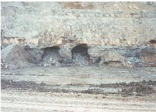
Photograph 4. Roof Falls and Web Collapse
