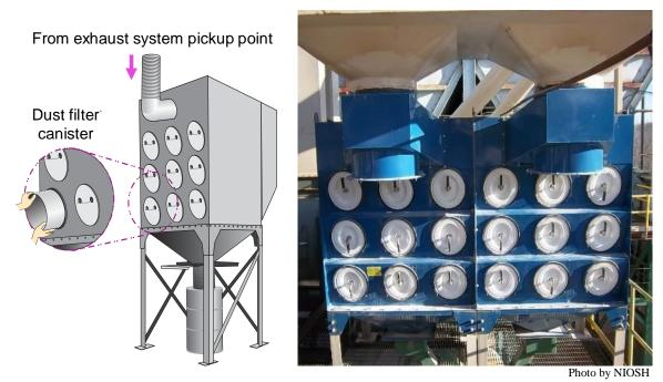
Figure 2.21. Cartridge collector with dust filter canisters. The left illustration shows a cutaway of a canister being replaced. The photo on the right shows a cartridge collector with the canisters mounted horizontally.
