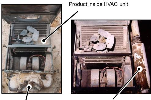
Damaged pre-filter canister
