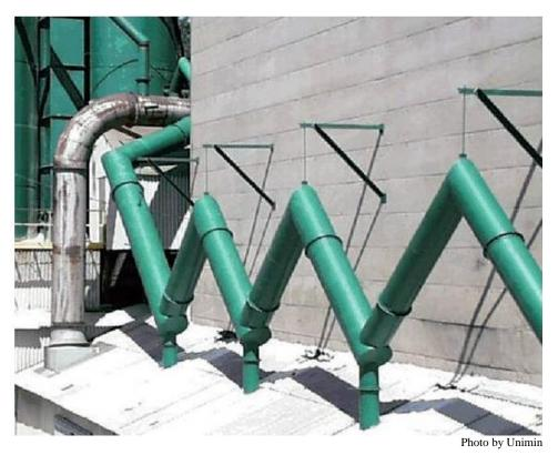
Figure 2.11. Sawtooth ("grasshopper") design of a low-velocity system with a drop-out duct back into the process at the base of each leg.
