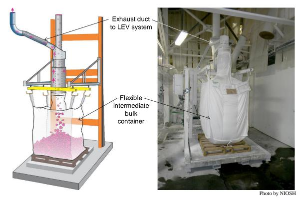
Figure 7.23. Illustration and photo of exhaust ventilation system being used during the loading of flexible intermediate bulk containers.
