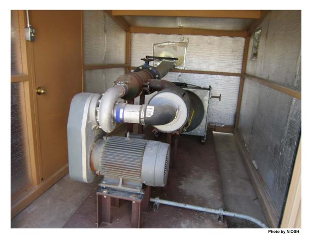
Figure A4. Permanent blower air supply system.
