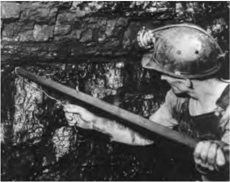
Figure 11. Miner preparing explosive shot in coal mine.
