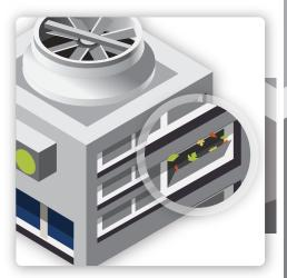
During weekly inspection of the cooling tower, Michelle discovers that leaf litter has accumulated in the reservoir.
