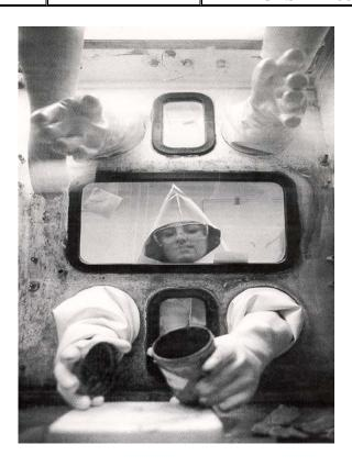
Figure 5 Other plutonium gloveboxes at Hanford. Note the viewing area in direct line with the lower torso in the center between the gloves. (2)
