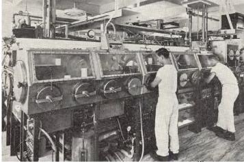
Figure 1 Plutonium gloveboxes at LANL<sup>(1)</sup>
