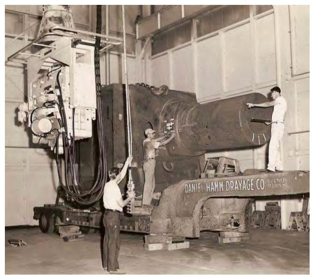
Figure 3. Betatron Radiography of the Axle of a Power Shovel Cast at GSI (Courtesy of [redacted])
