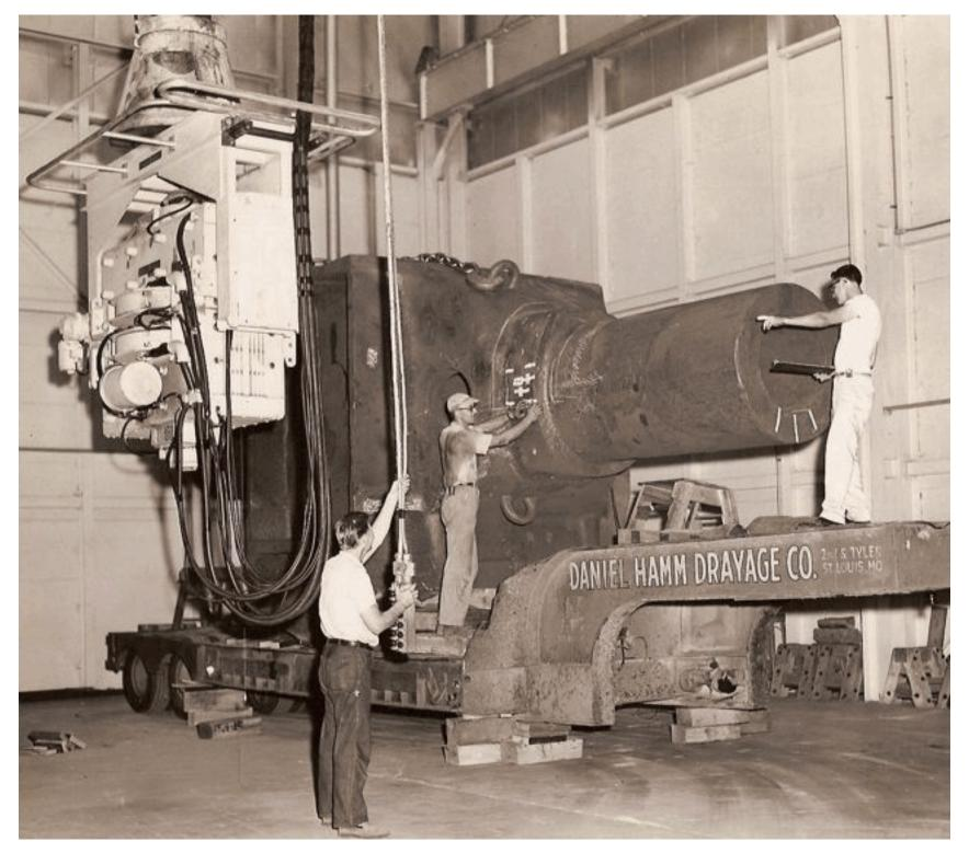
Betatron Radiography of the Axle of a Power Shovel Cast at GSI
