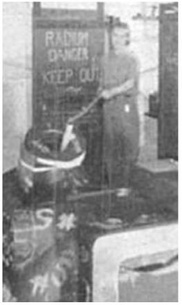
Source Being Removed from its Shield ("pig")
