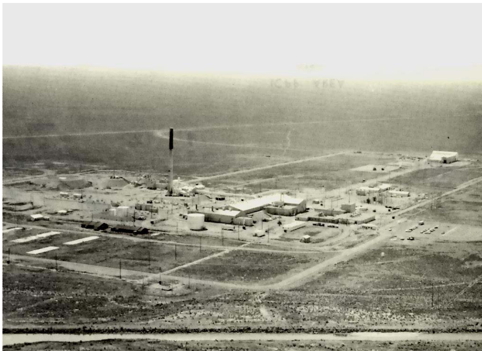
Figure 6. Aerial view of the Idaho Chemical Processing Plant (ICPP) at the INEEL. Fuel was received at the building in the upper far right and transported to the main process and laboratory building, the long white building in the center. The 250-ft (76.2-m) stack can be seen just to the left of center.
