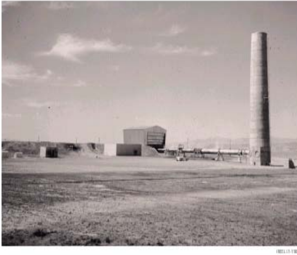
Figure 2-4 150-foot Exhaust Stack
