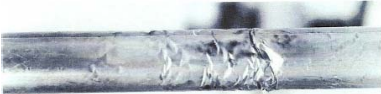
Figure 2-9 Insulation Liner Showing Wrinkling
