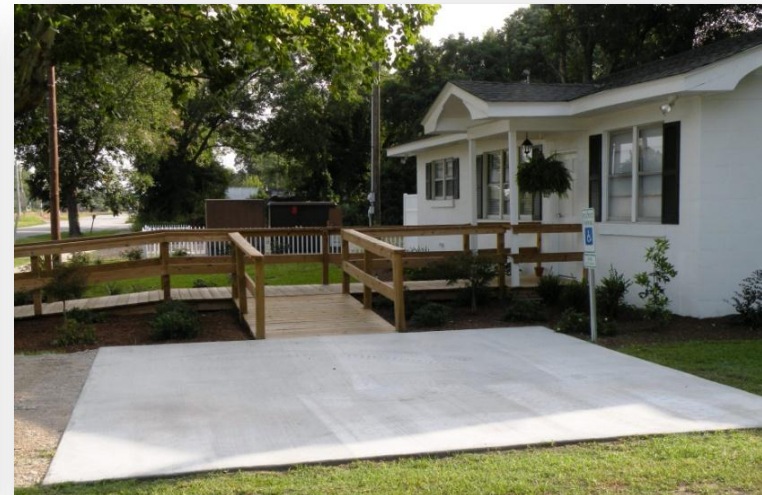
AFTER: Accessible parking with signage and easy slope to the ramp
