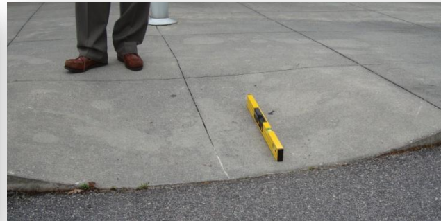
Measuring slope of curb cut from parking area to facility entrance
