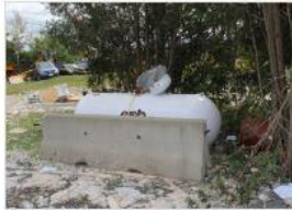
Propane tank involved in the explosion described in the FFFIPP Investigation Photo courtesy of Maine Fire Marshal
