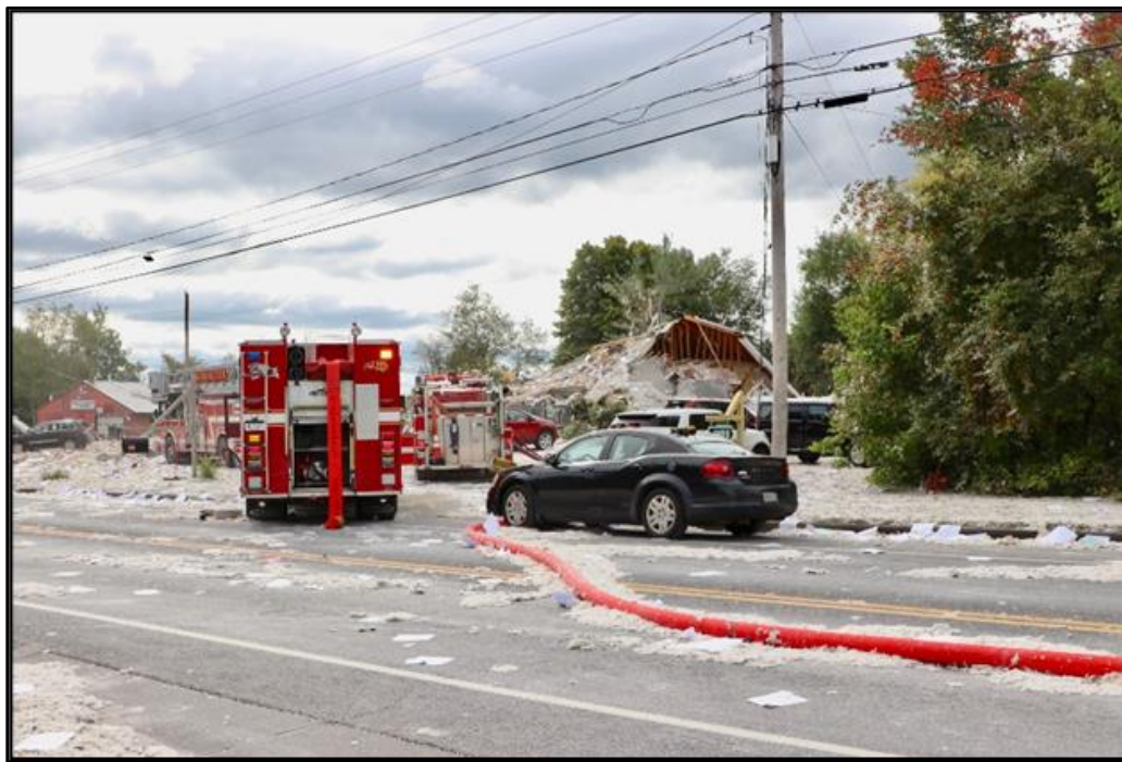
Destruction of the propane explosion. This photo shows Side Alpha/Side Delta of the building. The white debris is insulation and papers from the building. (Photo courtesy of the Fire and Rescue Department)
