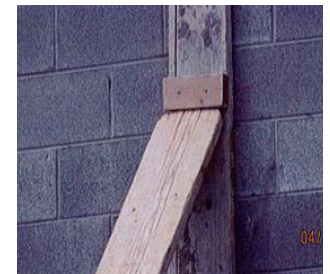
Interior Wall Bracing (Photos courtesy of TOSHA)
