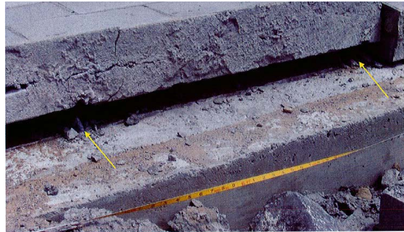
East Wall Rebar Location (Photo courtesy of TOSHA)
