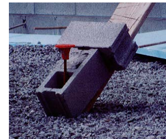
Interior Wall Bracing (Photos courtesy of TOSHA)
