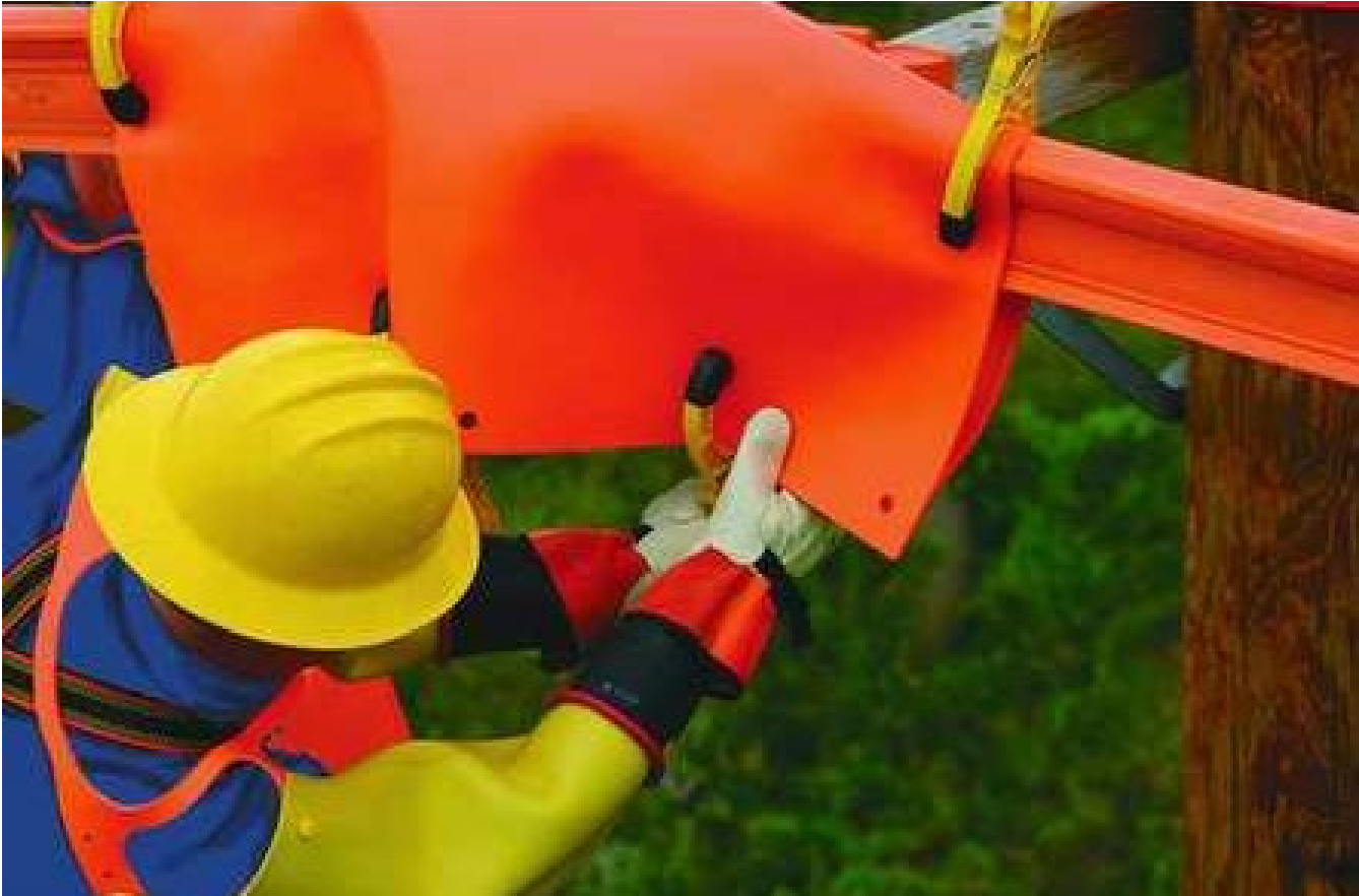
Image 8. Salisbury Insulating Blanket . (Zoro, 2023.)
