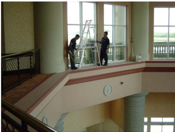
Figure 5. Close up of maintenance workers setting up for an atrium maintenance activity representing a serious fall hazard risk. A design that incorporates guardrails or built-in anchors for use with fall harnesses would substantially reduce this hazard.
