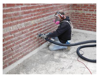
Figure 5 – Cyclone sampler in the breathing zone (NIOSH photo)
