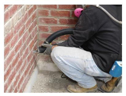
Figure 4 – Removing mortar in an inside corner (NIOSH photo)
