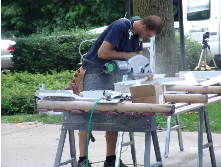
**Figure 3 – A worker (cutter) cutting fiber-cement siding using a prototype circular saw with a built-in cyclone dust collector and an air filter (“red-spur saw”). Photo courtesy of NIOSH.**
