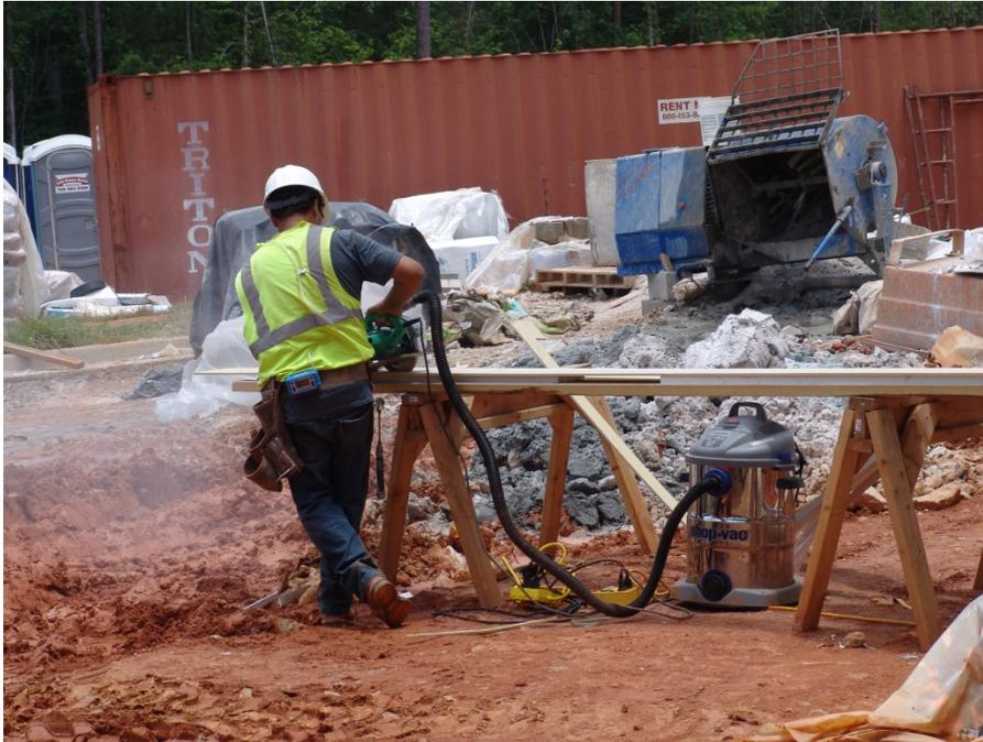
**Figure 2 – A worker (cutter) cutting fiber-cement siding using a dust-collecting circular saw that was connected to a shop vacuum.**
