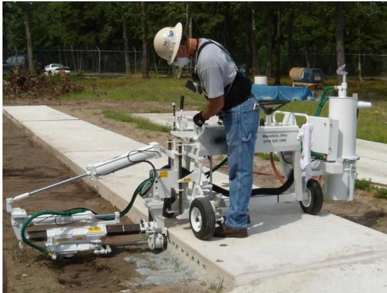
Figure 1 – Laborer Operating Dowel Drill
