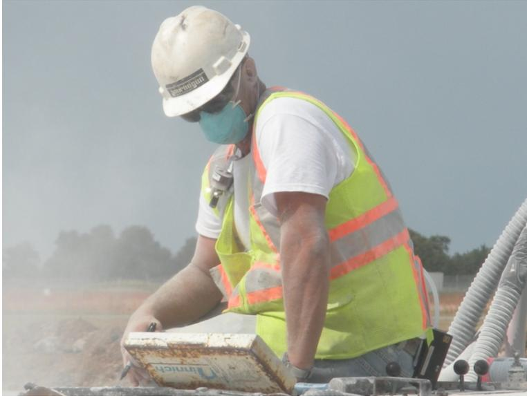
**Figure 3 - Sampler in Worker's Breathing Zone and Pump at his Waist**
