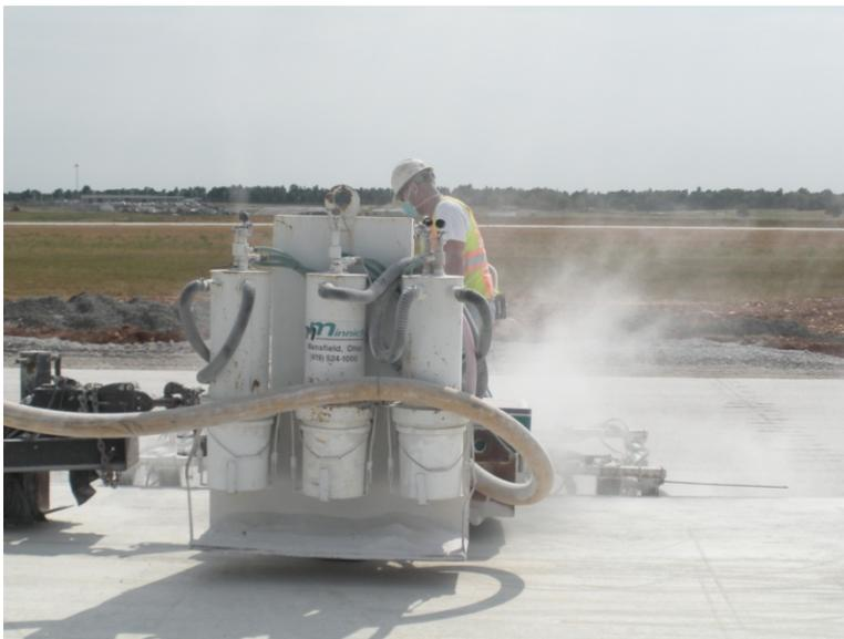
**Figure 8 - The Flexible Duct Forms a Loop When it Changes Direction. Note the Hose Connected to the Left Side of the Dust Collector on the Right.**
