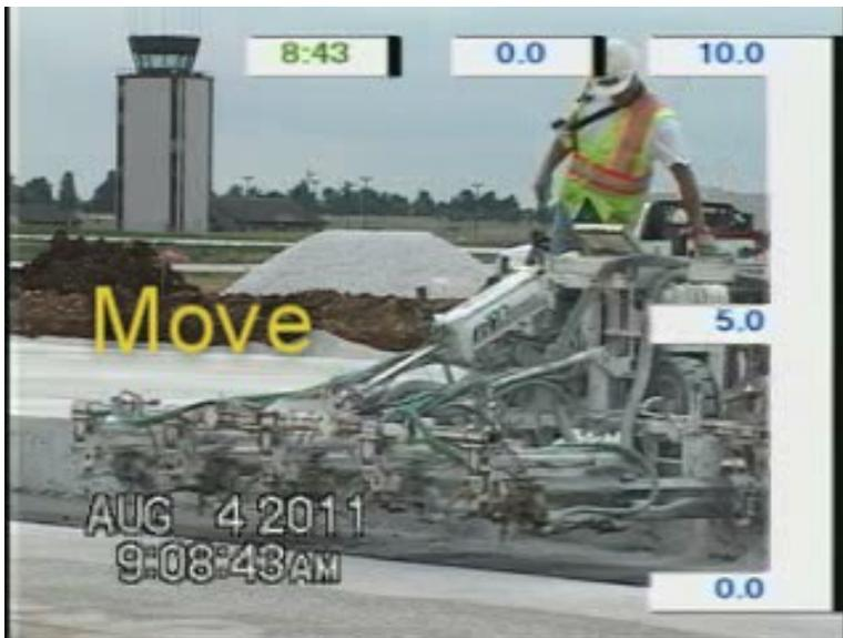
Figure 12 - Moving the Drill Did Not Result in a Spike in Respirable Dust Exposure
