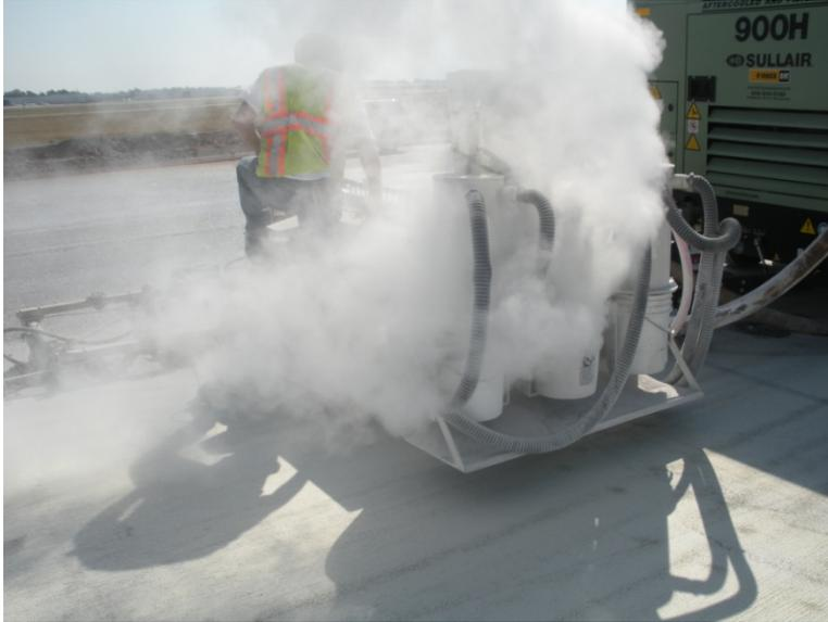
**Figure 9 - Purging Creates Clouds of Dust**
