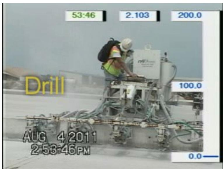
Figure 13 - The Drilling Task Did Not Result in a Spike in Respirable Dust Exposure
