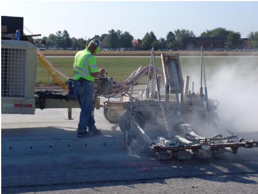
Figure 1 - Laborer Operating a Minnich Dowel Drill
