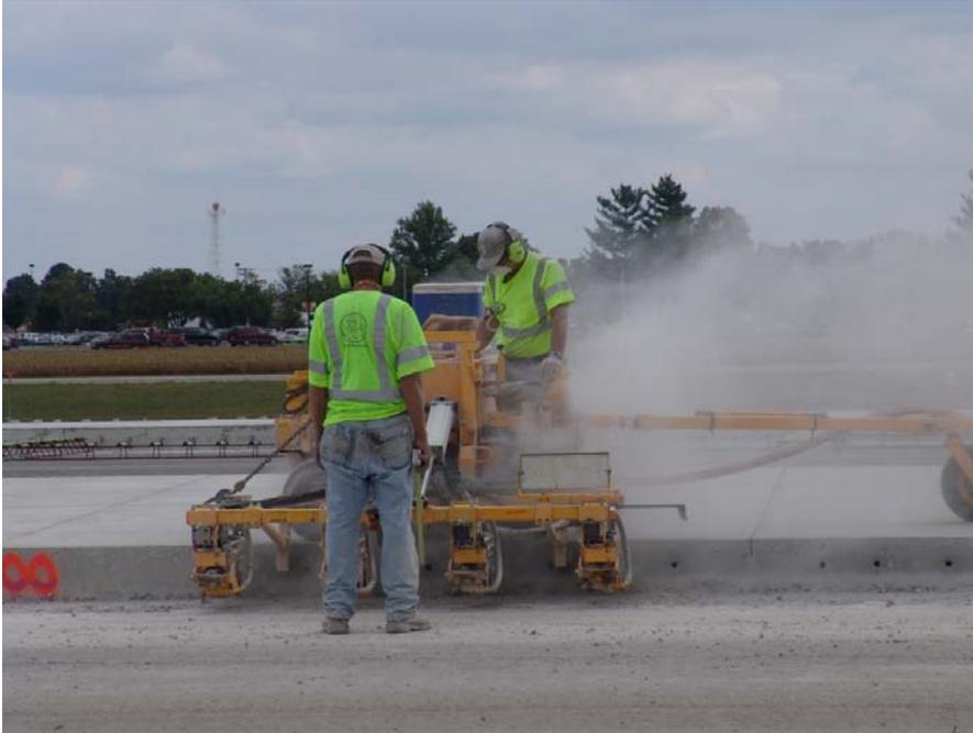
**Figure 2 - Laborer Operating an E-Z Drill Dowel Drill**
