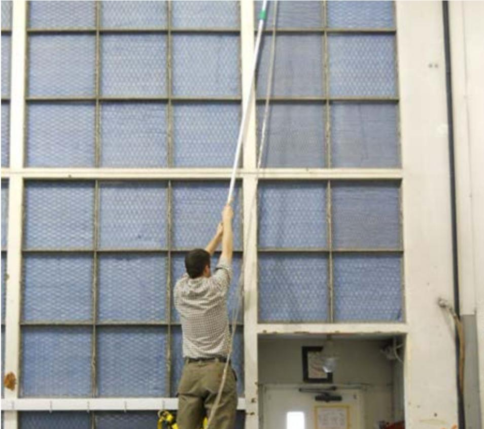
Figure 3. NMCSD industrial hygienist measuring supply air velocity, using extension pole to reach high on the filter.
