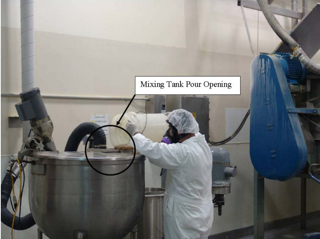
Figure 5. Large mixing tank exhaust hood.
