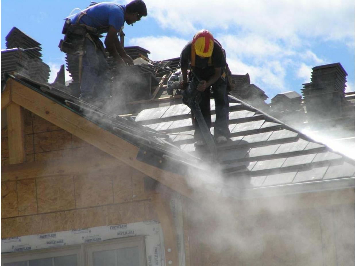
Figure 4. Workers using leaf blower to clean dust from tiles.
