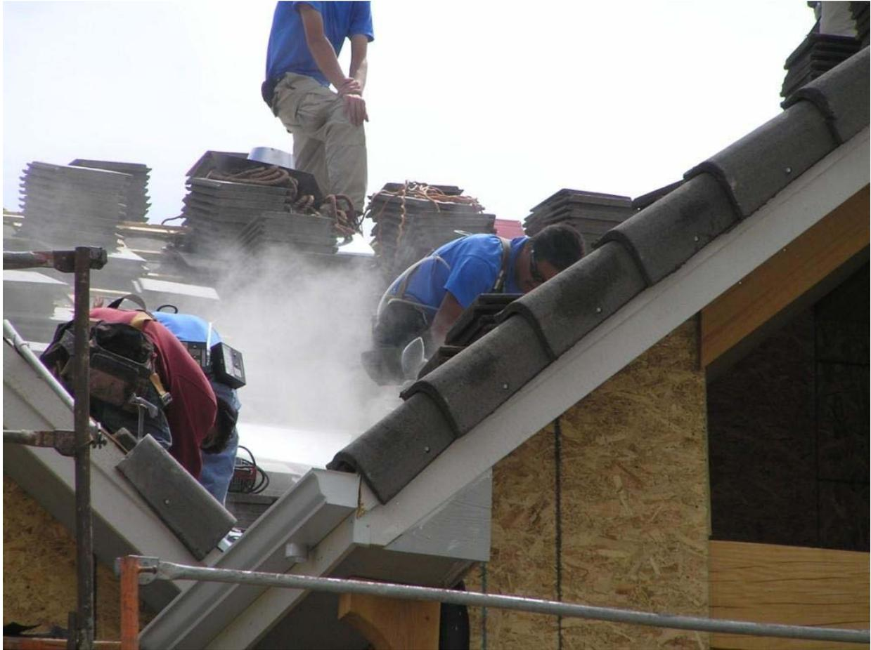
Figure 5. Workers cutting concrete roofing tiles.
