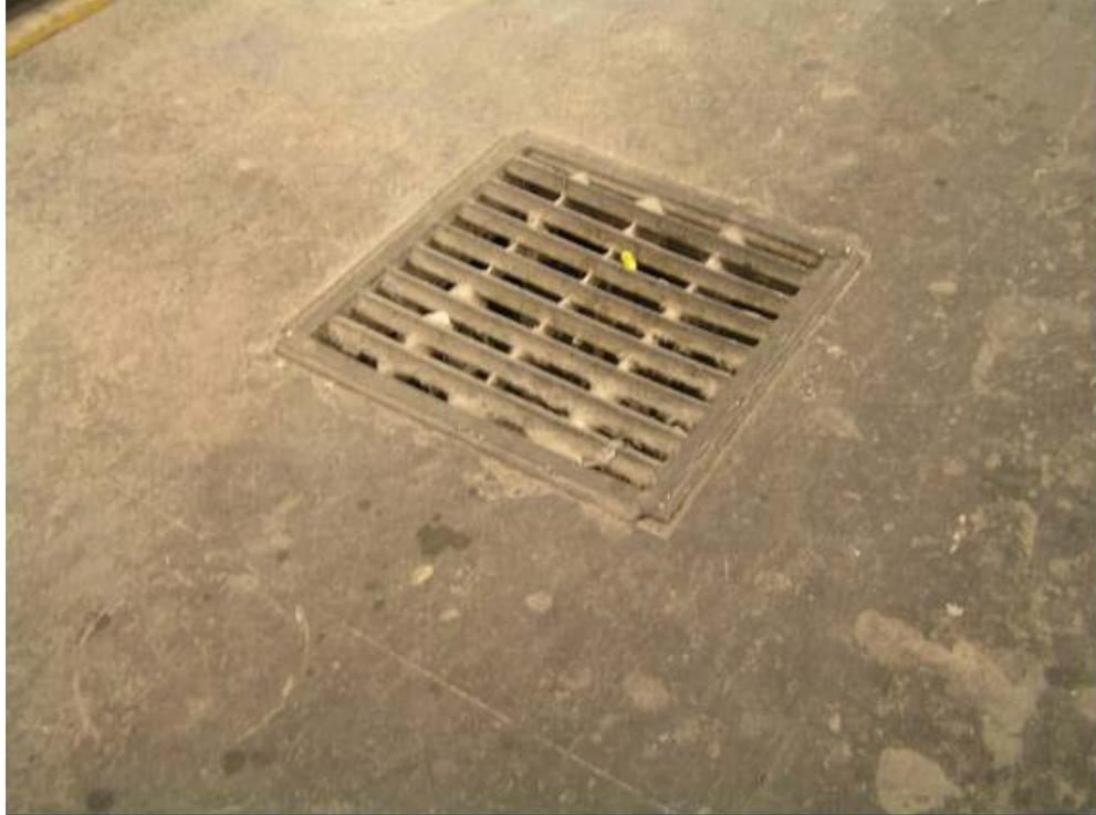
**Figure 5:** In-floor exhaust ventilation in the L Building
