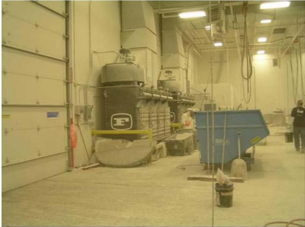
**Figure 4:** Exhaust ventilation in the web cut and trim area of the M Building
