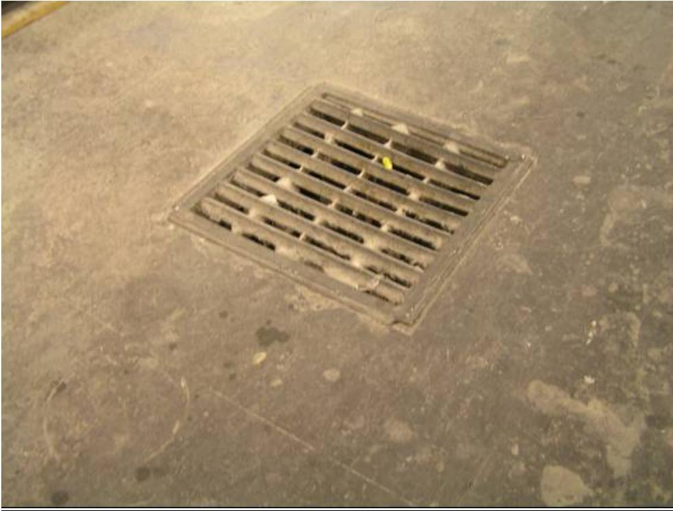
**Figure 3:** In-floor exhaust ventilation in the L Building
