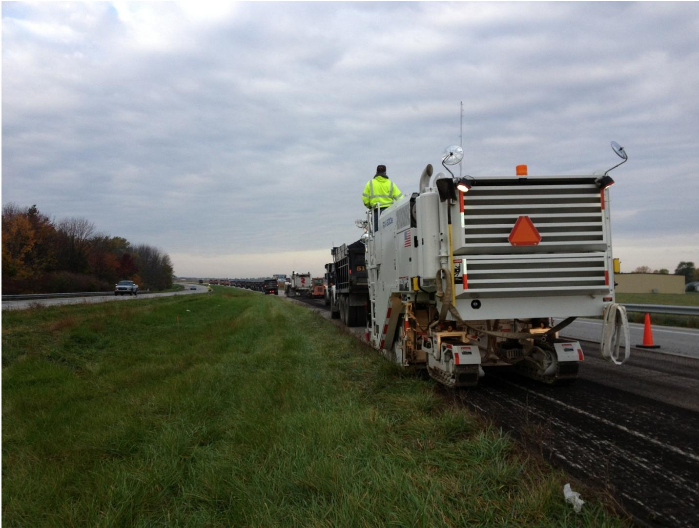
Figure 1: Evaluated milling machine with local exhaust ventilation system
