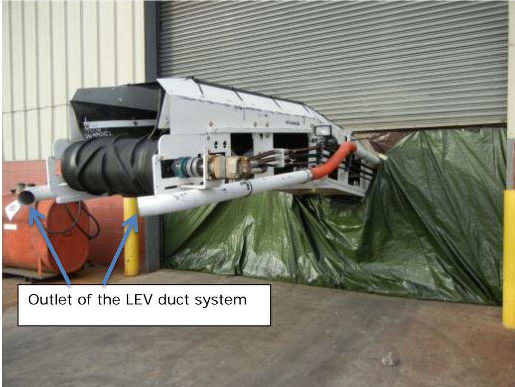
Figure 2: Outlet of the LEV system through the overhead door
